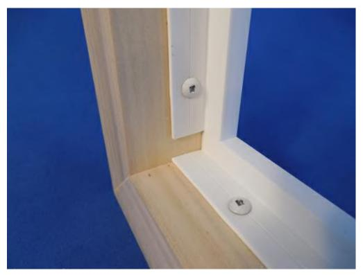
"Inside" the opening with butt corner installation: Top and bottom extrusion (widths) are always sized to be the full opening. Heights are cut to fit in between the width extrusions. The gap shown in the photo left is normal and notching of the height extrusions is not required.
