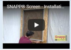
SNAPP® Screen System Installation Series - Part 3 reviews the technique and process for installing screen material into the SNAPP® Screen System screening extrusion
