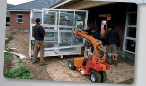
The wide tires make the lifting device suitable for difficult off-road jobs.
